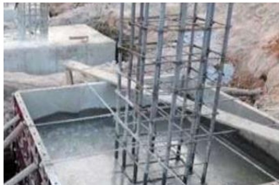
Gambar 3. 2 Pondasi Telapak [2]
