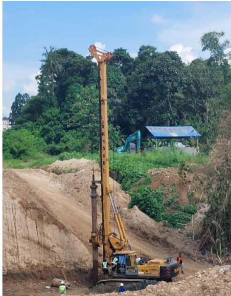
Gambar 4. 4 Drilling Rig, XCM6-XR150DII [11]
