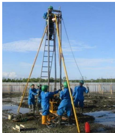
Gambar 3. 10 Pondasi Bored Pile Gawangan [8]
