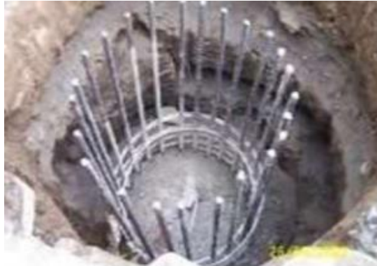
Gambar 3. 8 Pondasi Bored Pile [5]
