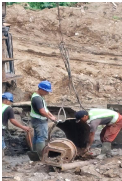
Gambar 4. 18 Proses Pengikatan Casing [11]
