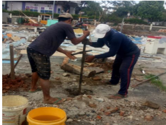
Gambar 3. 11 Pondasi Bored Pile Strauss Pile [8]
