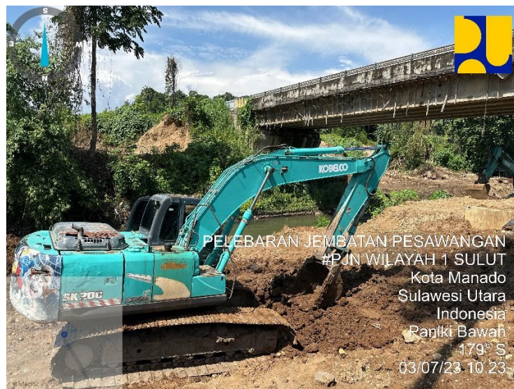
Gambar 4. 3 Excavator Kobelco SC 200 [3]
