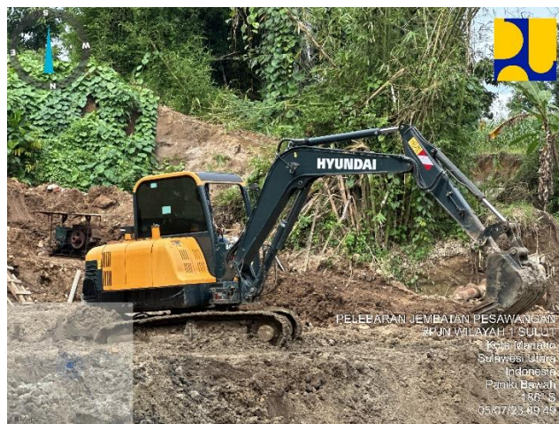
Gambar 4. 2 Excavator Hyundai Robex 75-7 [3]
