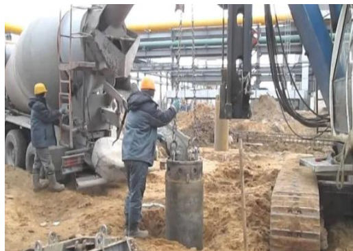
Gambar 3. 4 Tiang pancang beton cast in place
