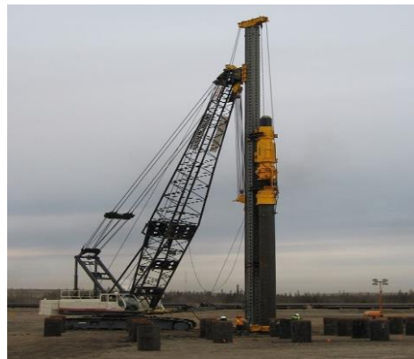
Gambar 3. 7 Drop hammer
