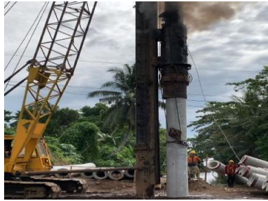
Gambar 3. 10 Diesel hammer
