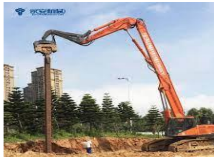
Gambar 3. 11 Vibratory hammer
