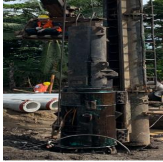
Gambar 4. 2 Diesel hammer
