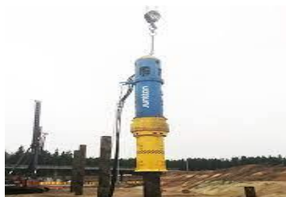
Gambar 3. 12 Hydraulic hammer
