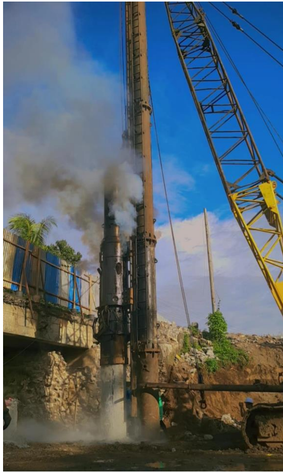
Gambar 3. 2 Diesel Hammer [4]
