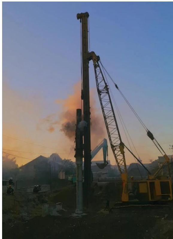
Gambar 3. 1 Alat Drop Hammer [4]
