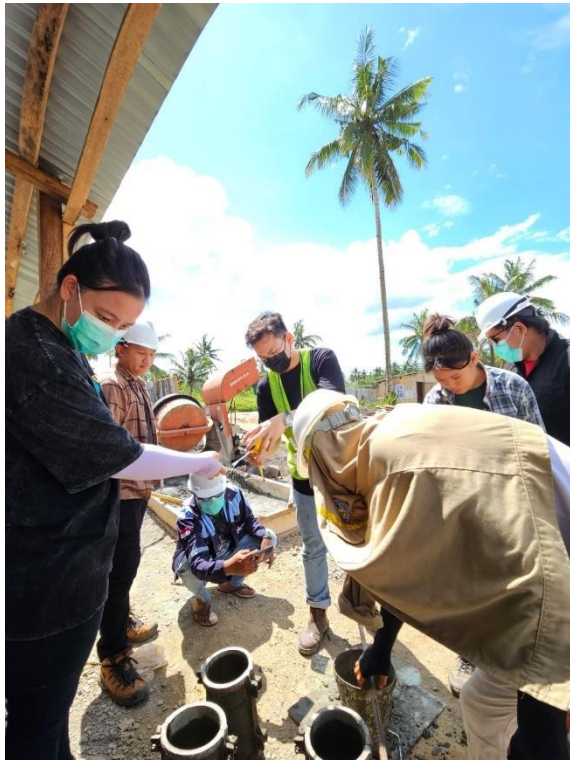
Gambar E- 1 Test Slump
