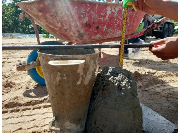
Gambar 4. 17 Uji slump 50m tahap II [5]
