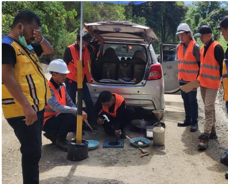
Gambar 4. 5 Proses Pengujian Sand Cone [2]
