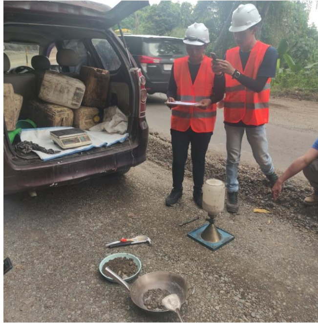
Gambar 4. 6 Proses Pengujian Sand Cone [2]
