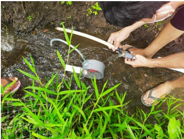
Figure 4.1. Hose Installation on Generator
